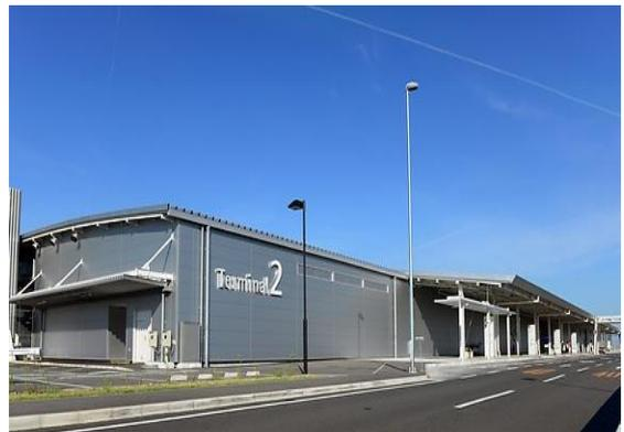
Peach Aviation requested that Terminal 2 have a simplified design in order to minimize operating costs. The terminal is a single-story building, thus eliminating the cost of elevators. Passageways to aircraft have no air conditioning. The terminal also has no boarding bridges, having 4 domestic, 3 swing, 2 international boarding gate. In case of rain, passengers are lent umbrellas to use as they walk to the aircraft.
