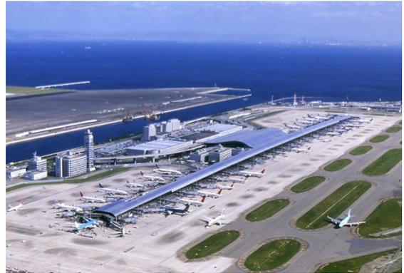
The terminal's roof is shaped like an airfoil. This shape is used to promote air circulation through the building: giant air conditioning ducts blow air upwards at one side of the terminal, circulate the air across the curvature of the ceiling, and collect the air through intakes at the other side.
