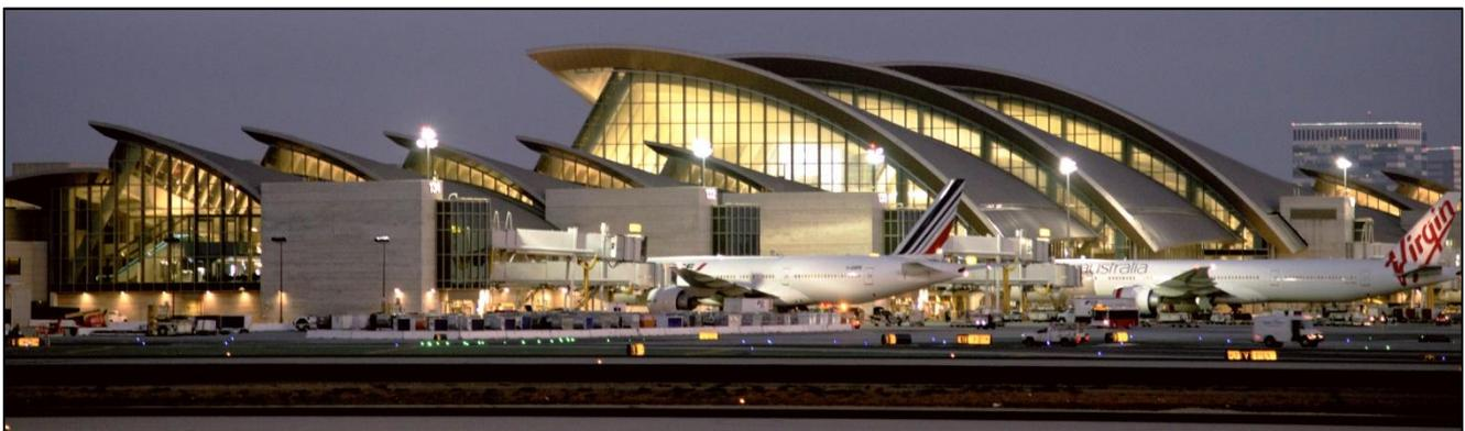
Nine of TBIT's 18 gates can accommodate the new-generation Category VI aircraft such as the Airbus 380 and Boeing 747-8 Intercontinental jets. A-380 aircraft are served by three passenger boarding bridges (one reaching an aircraft door on the upper deck) for efficient boarding and deplaning. Each gate is equipped with a Safegate Advanced - Visual Docking Guidance System.
